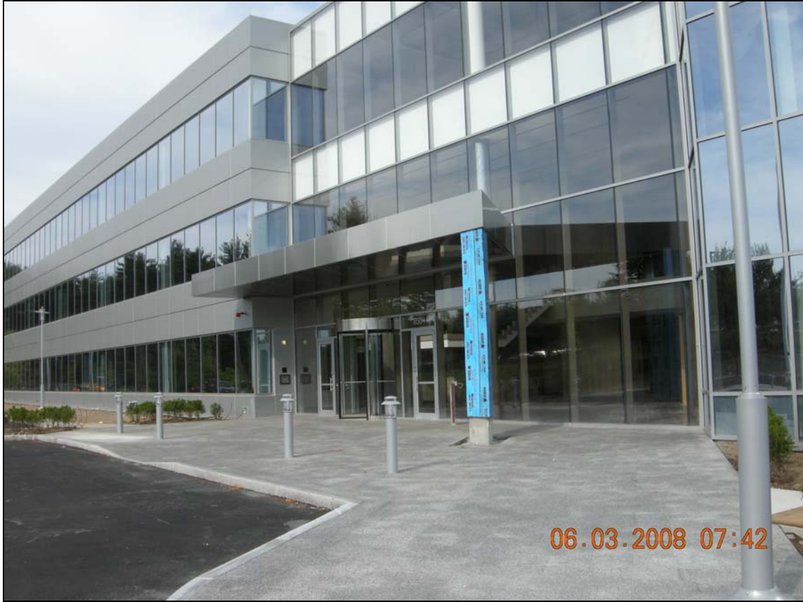
View of South Main Building Entrance with Two Story Atrium During Construction
