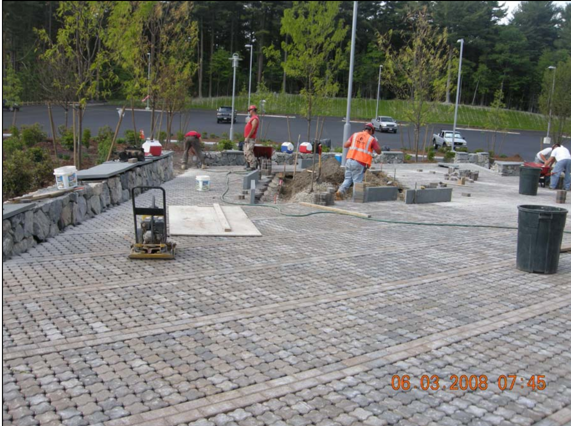
View of Future Outdoor Eating Area During Paving Operations
