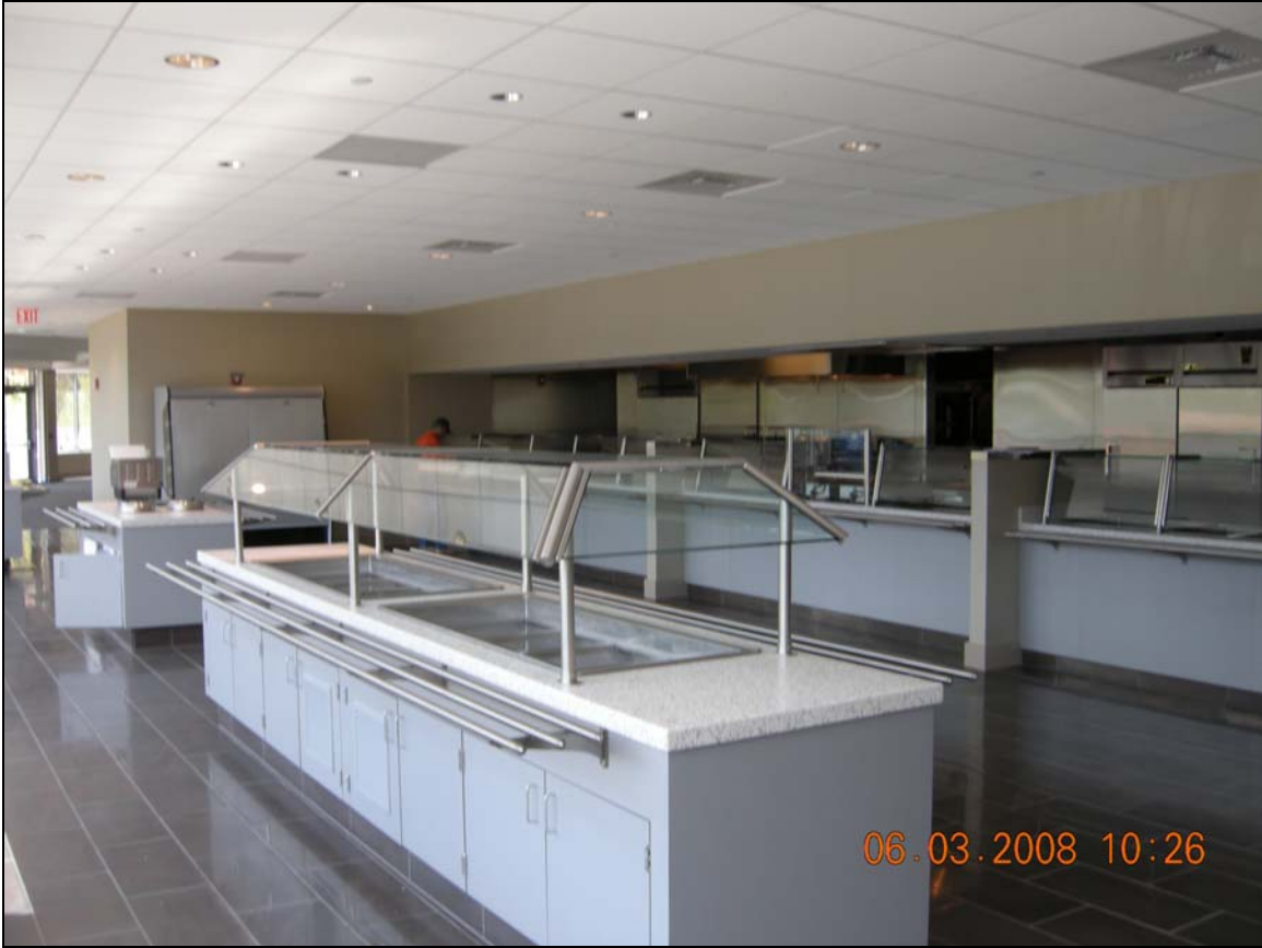
View During Construction of Employees Cafeteria
