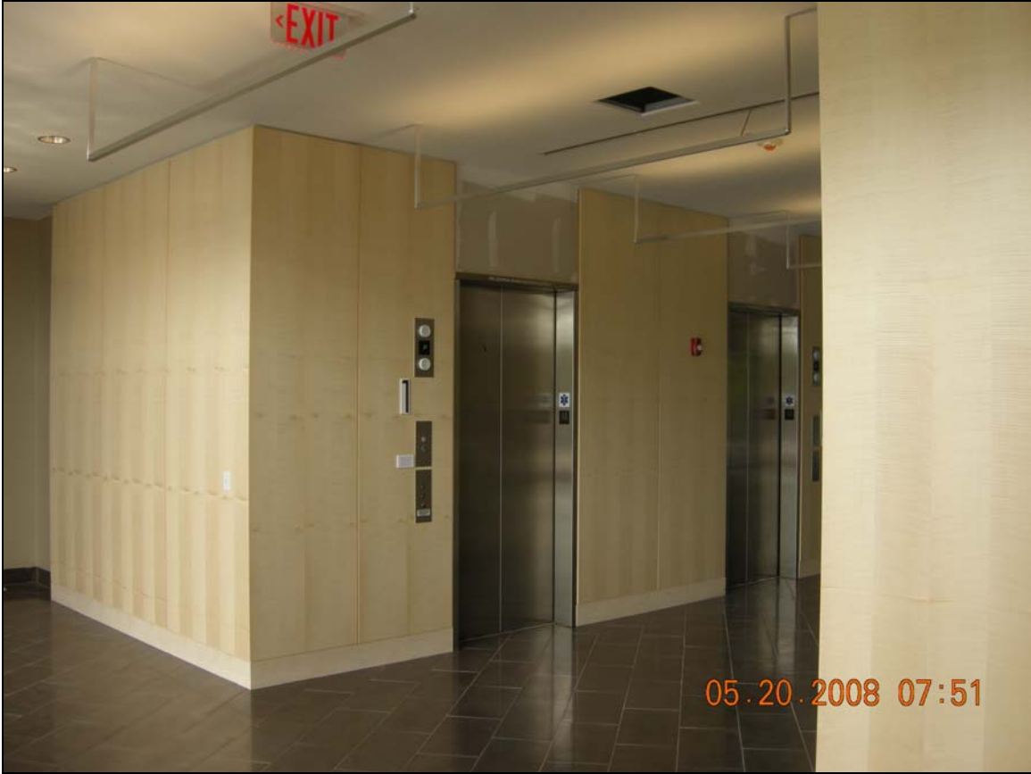
View of Elevator Core Finishes – Veneer Wood, Stainless Steel & Tile Floors
