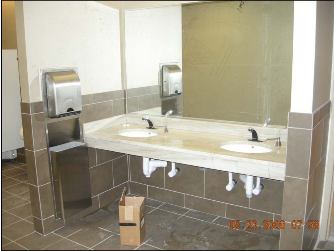
View of Public Toilets During Construction
