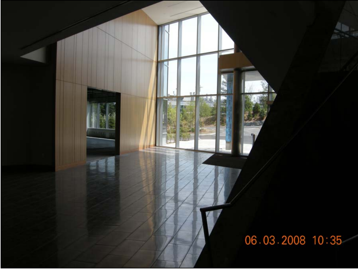
View of Two Story Atrium During Construction
