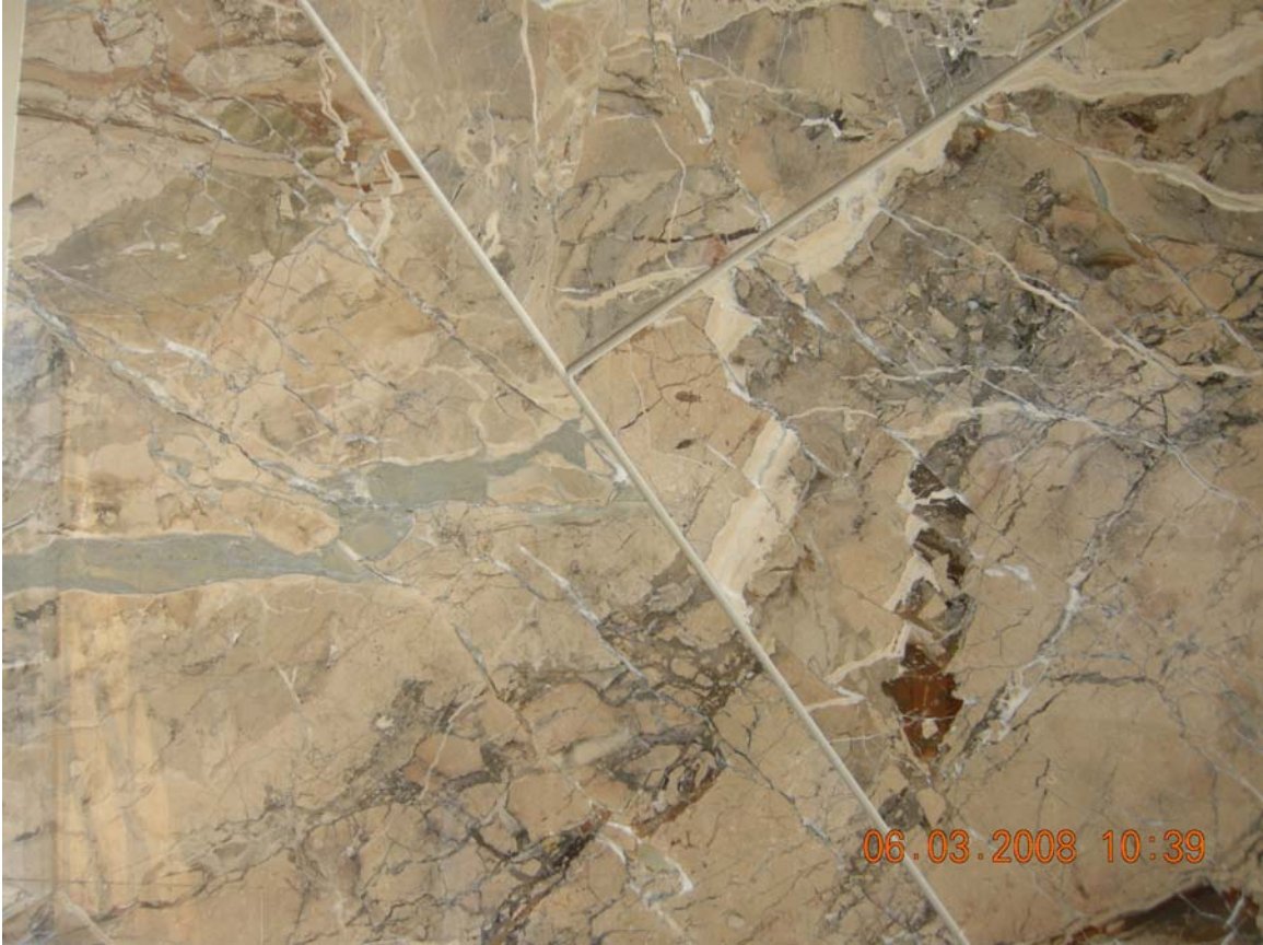
View of Stair Detail at Stone Veneer
