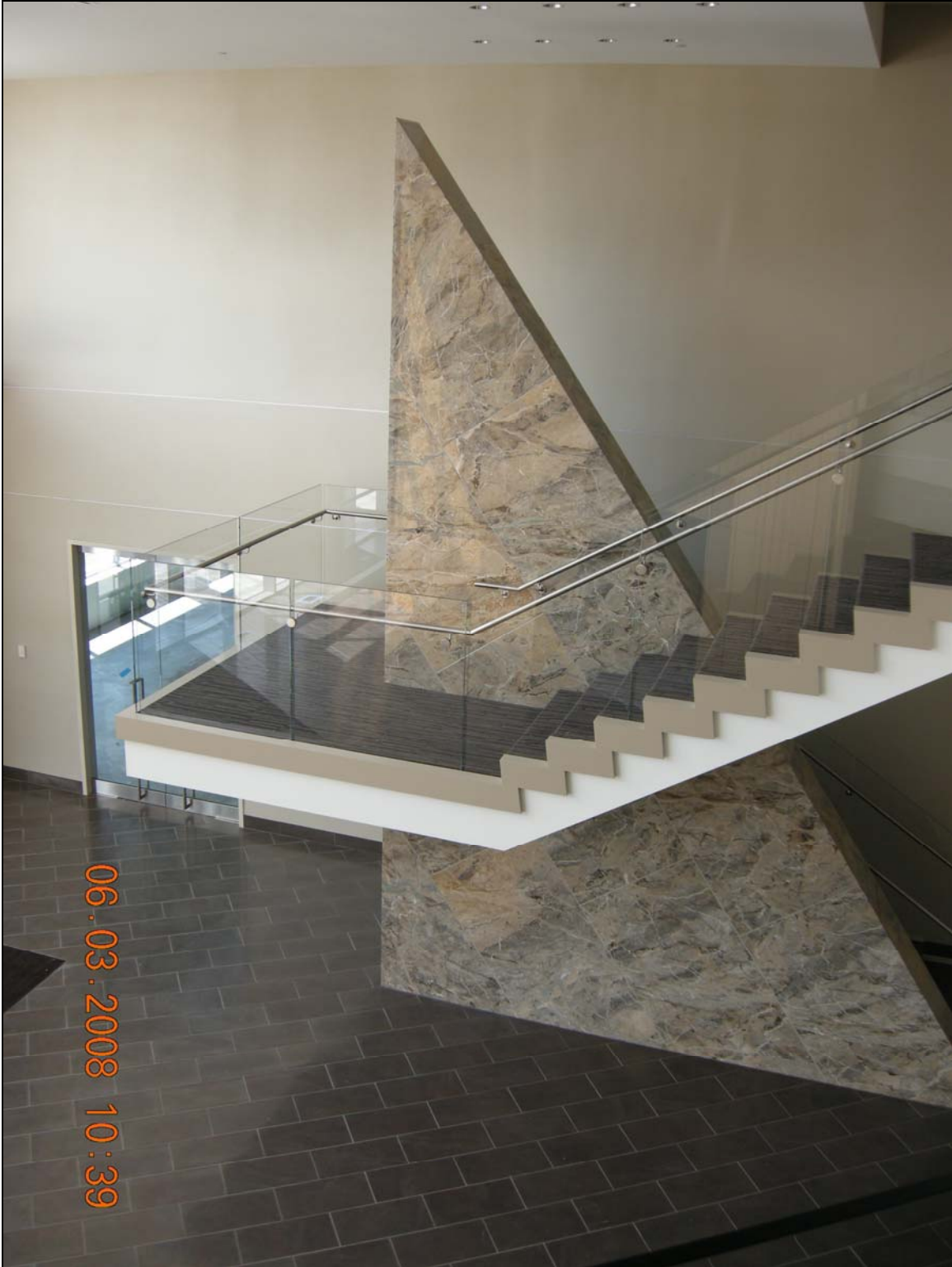
View of Stair in two Story Entry Atrium
