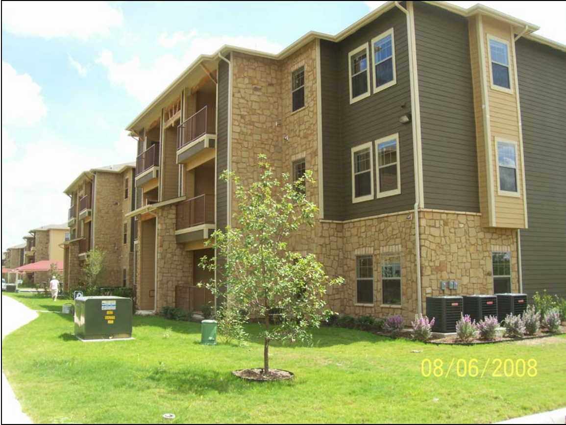
View of Typical Apartment Balcony, Landscaping & Car Ports
