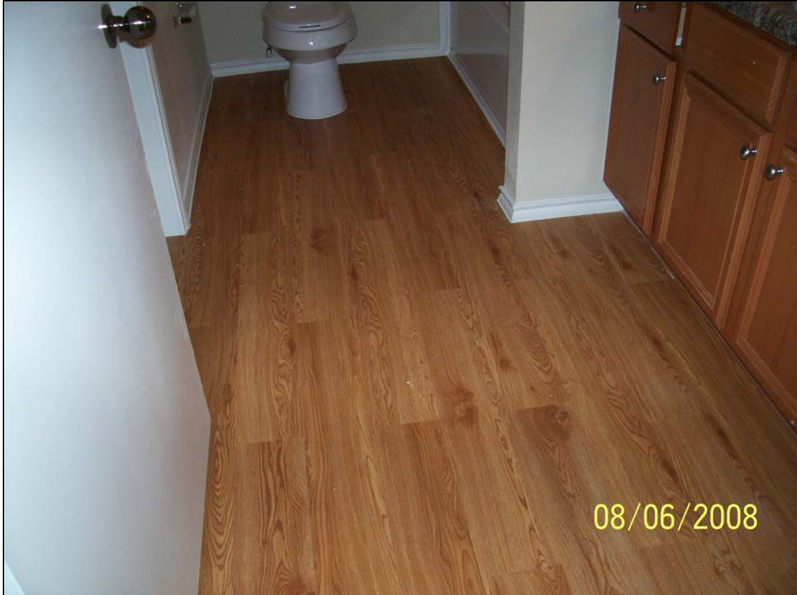
View of Typical Bathroom Floor Finish
