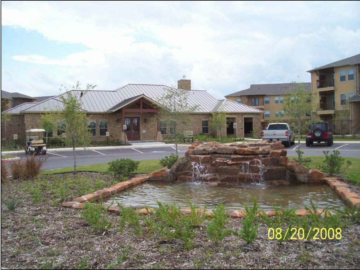
View of Club House-Leasing center from Entrance to Property
