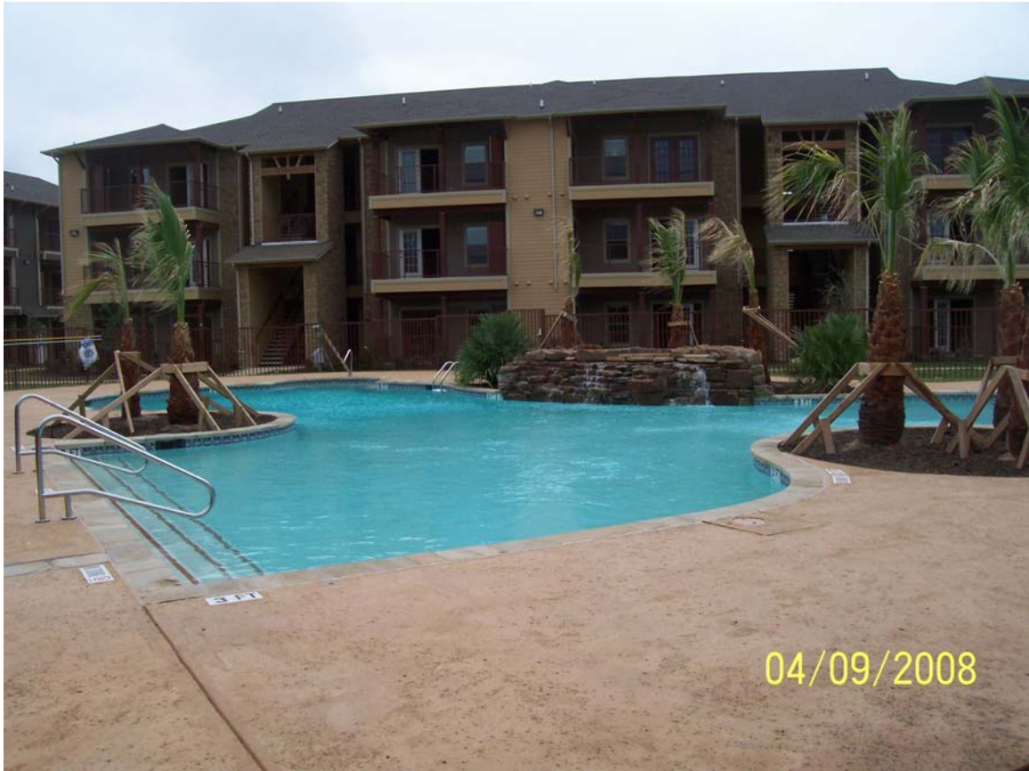
View of Outdoor Swimming Pool During Construction & Landscaping
