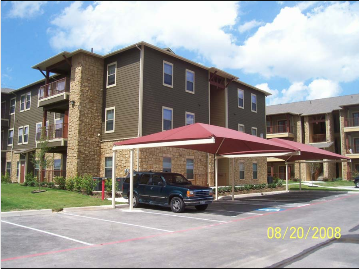
View of Typical Building Façade with Stone Veneer Accent
