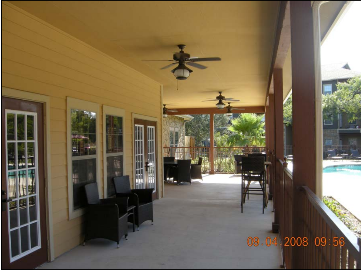
View of Club House & Pool Covered Porch
