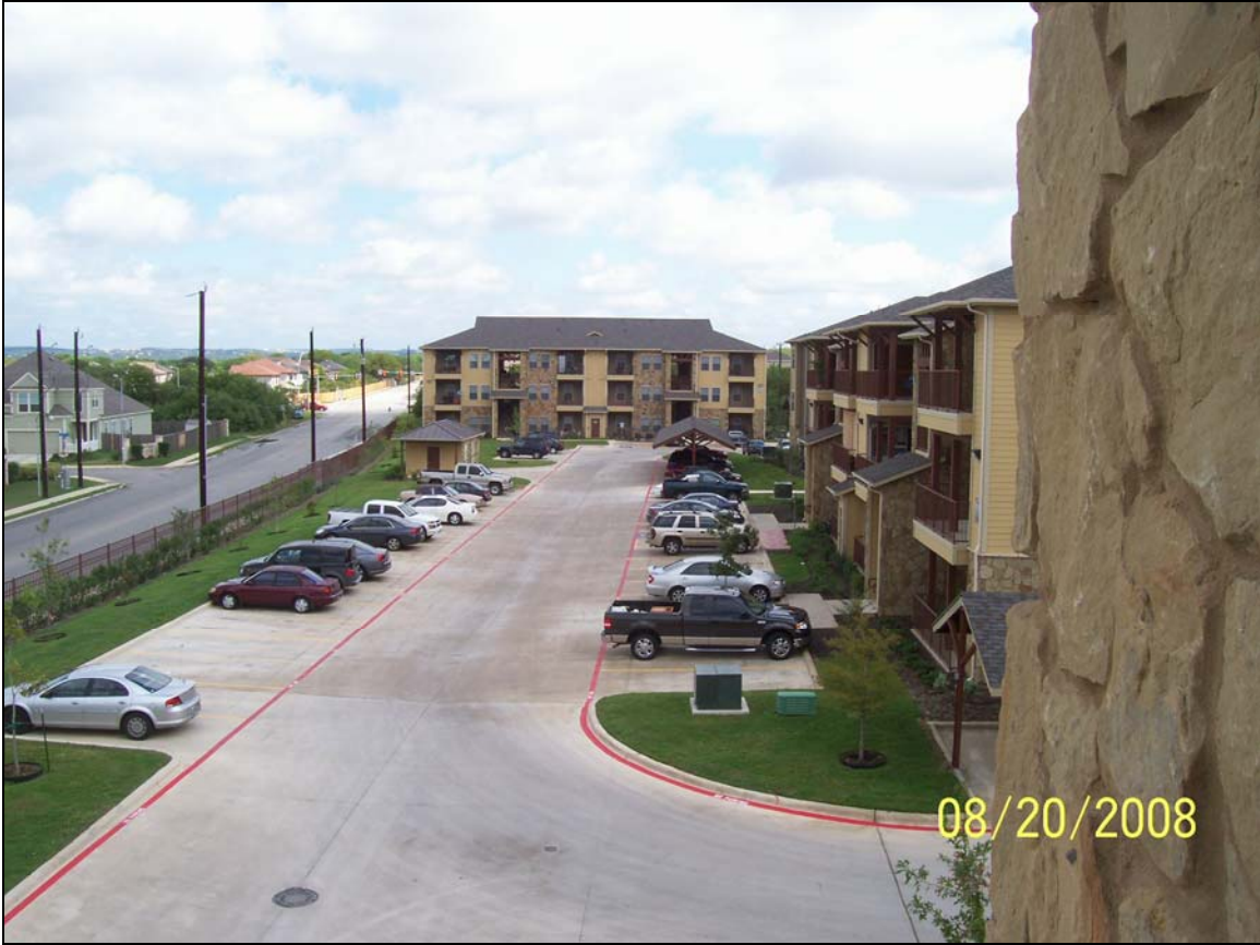
View of Typical Building Facades
