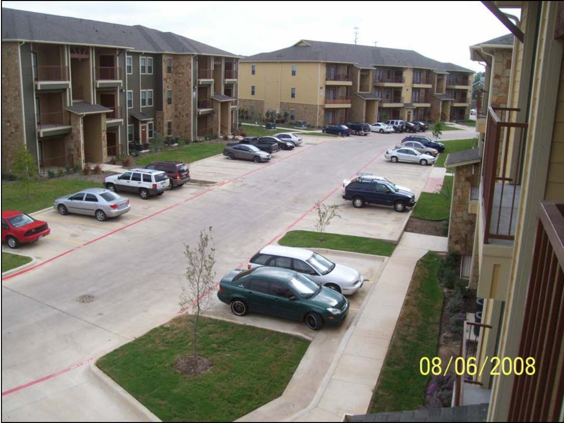
View of Typical Building Facades
