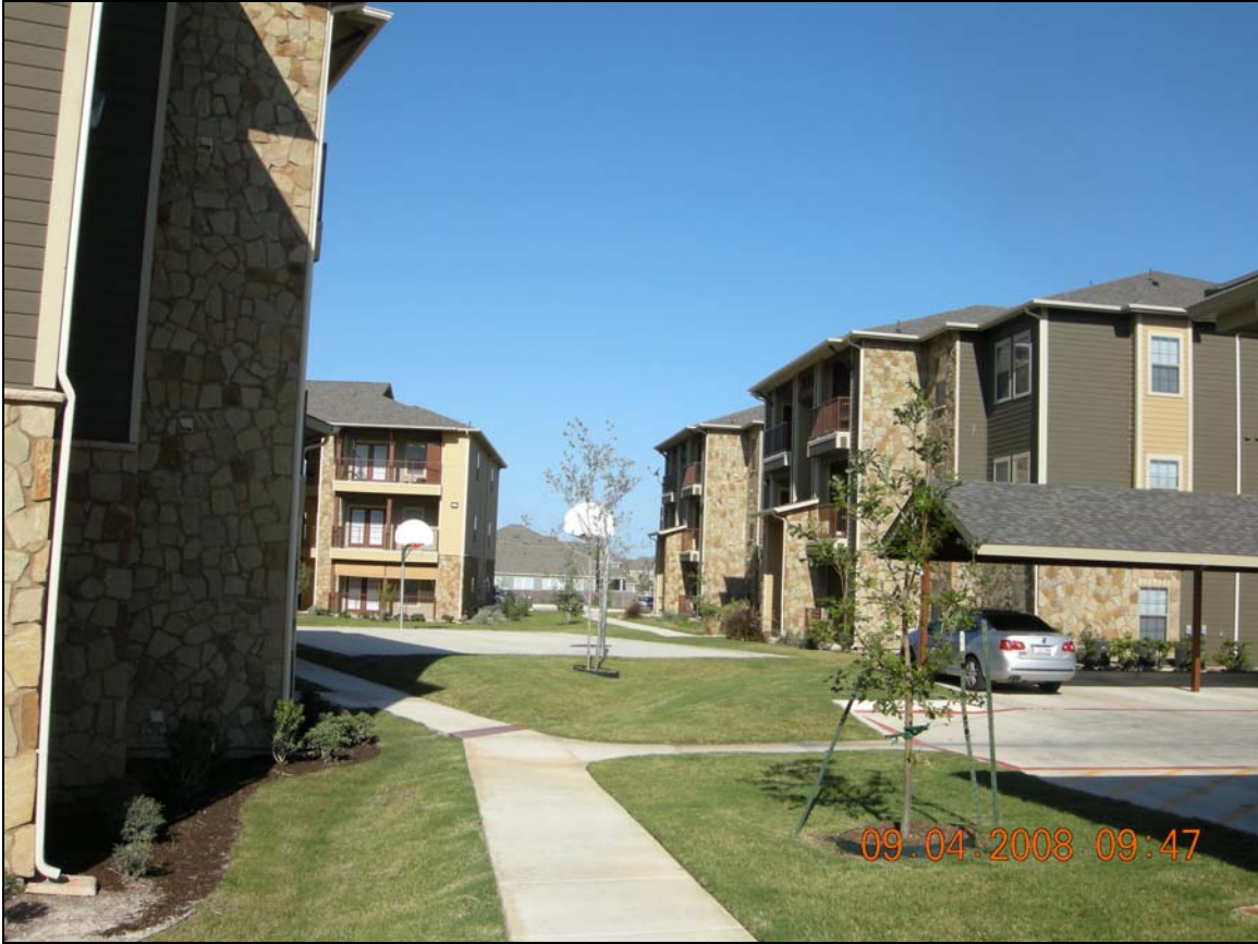
View of Typical Building Facades, Landscaping & Carport
