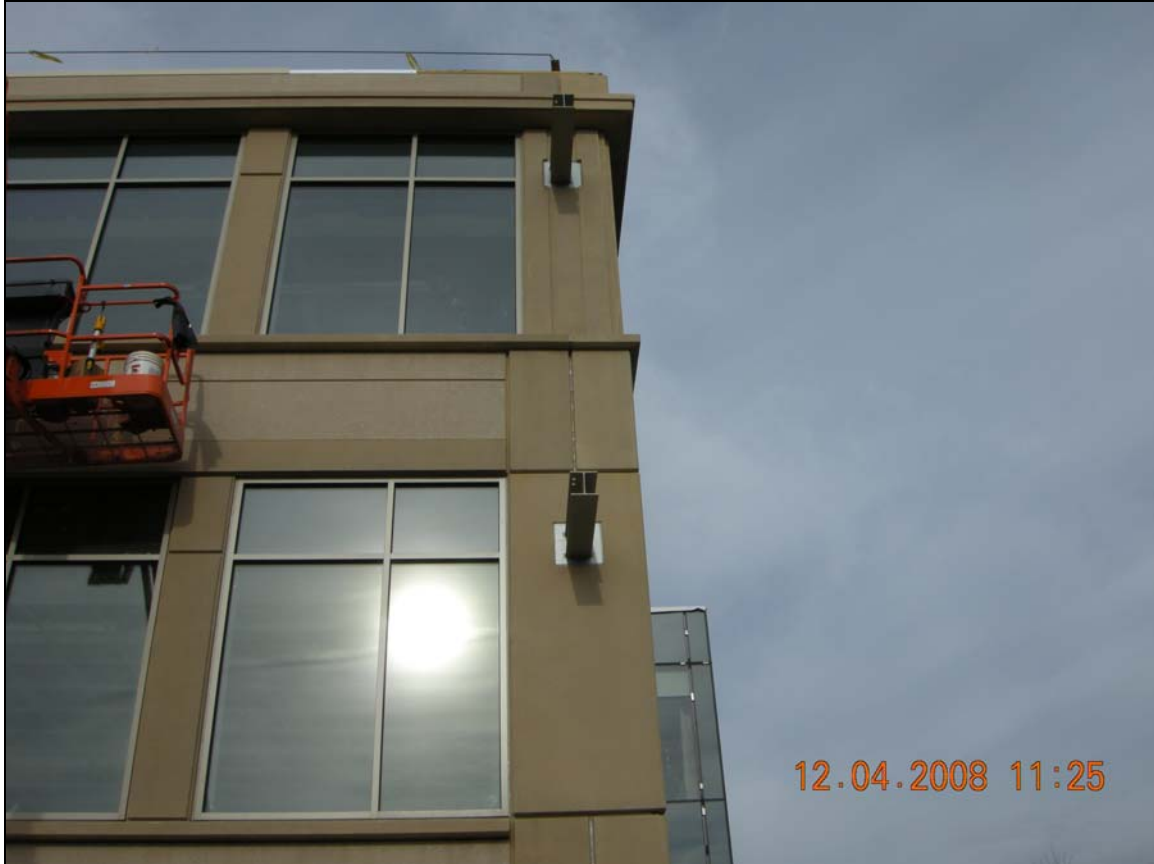
View of Outrigger Supports for Sunscreen Louvers on South Facing Facades
