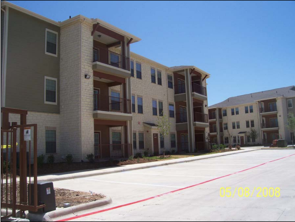
Project Consists of Eleven Apartment Buildings
