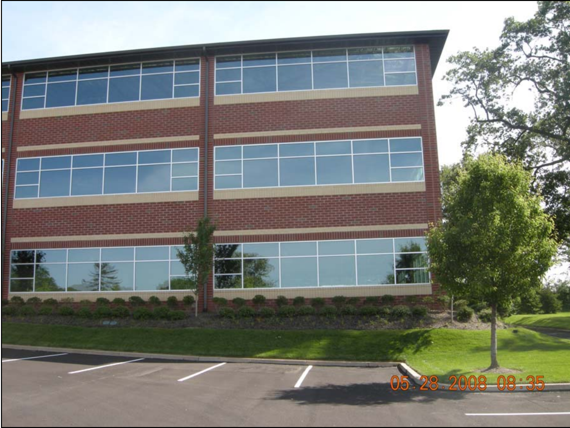
View of Three Story Building Façade – Typical Exterior Materials / Pre-fabricated Brick-Pre-cast Concrete Panels + Alumn. Windows
